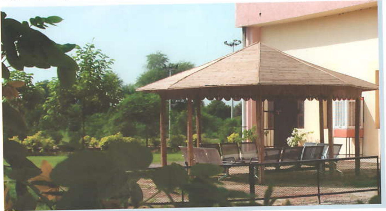
A Bamboo Hut close to the Canteen-cum-Mess
