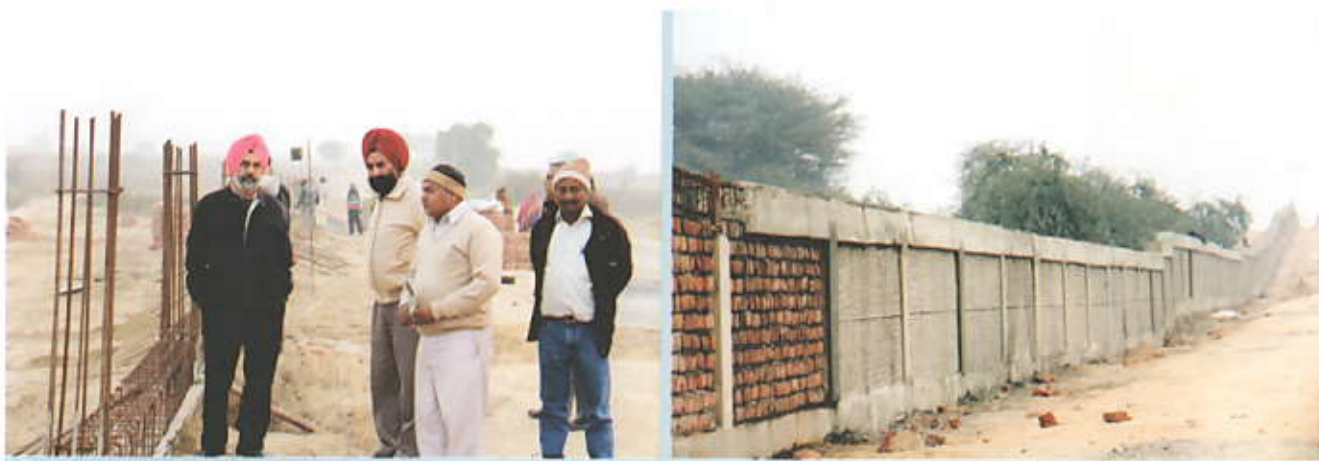
Under construction boundary wall of the Main Campus of the University
